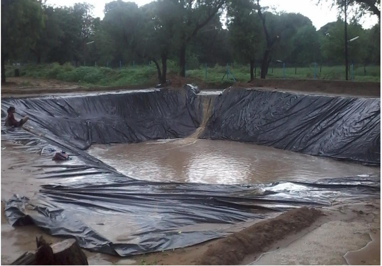
Water Harvesting through Rain water collection in Farm pond at the Institute
