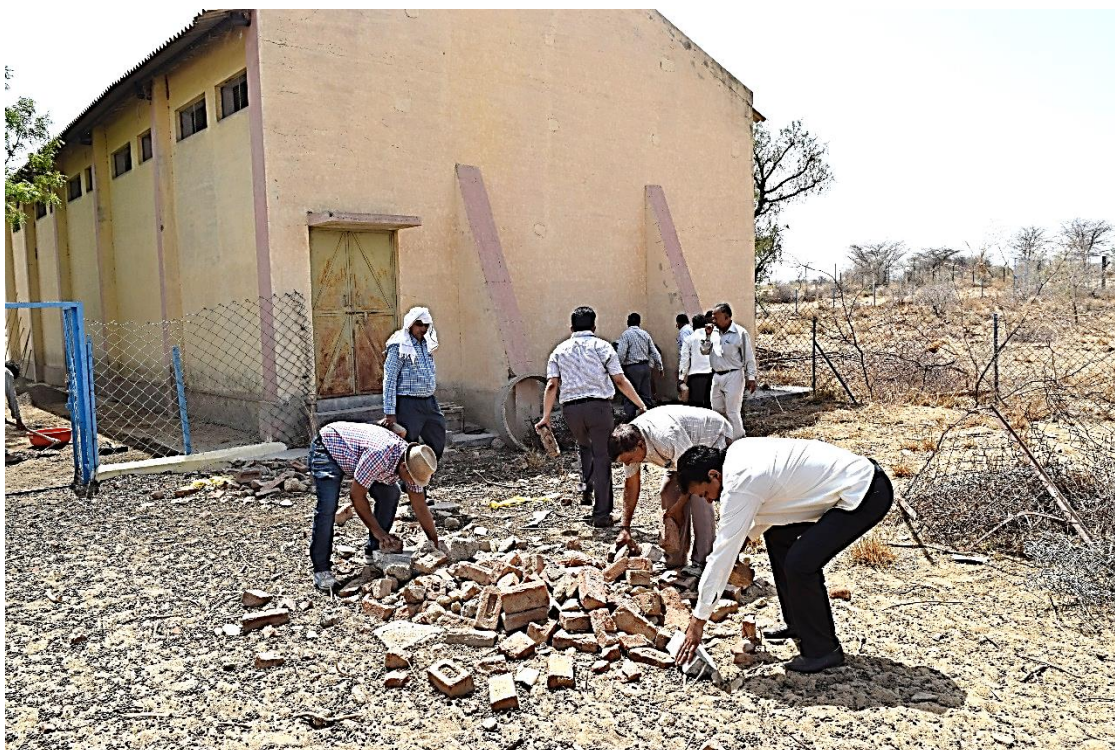
Cleaning and relocating the debris
